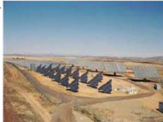
Over 1.5 MW of HCPV system is under construction. These systems use plastic lenses to concentrate the sunlight 250 times onto much smaller, high efficiency solar cells. This reduces the area of PV material by 250 times, which should result in a potentially low cost solar electric generation technology.
